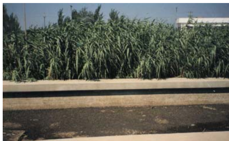
Photo 13: Reed bed after overcharging
