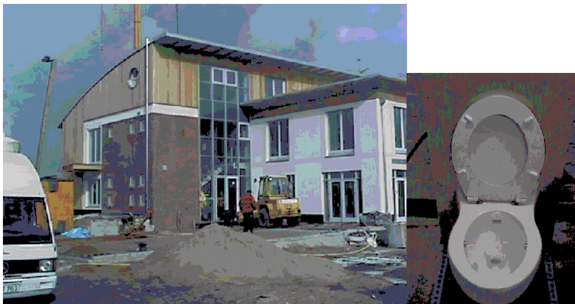
Figure 4: Community building of settlement 'Flintenbreite' for 350 people containing vacuum pumping station, biogas plant and combined heat and power generation, detail: vacuum toilet flushing with around 1 litre of water.
